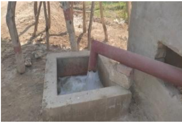
Figure 3: Tile Drainage System installed at Nawazabad
