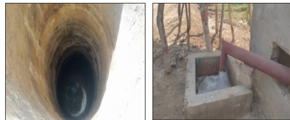
Functional Tile Drainage System
