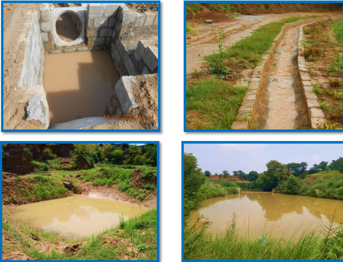
Figure 30: Stormwater harvesting at the farm
