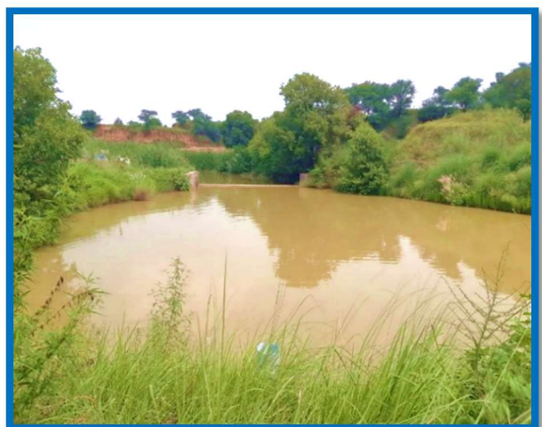
After filling the pond with rainwater
