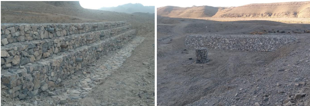
Figure 20: Leaky dam structure in Balochistan (left) and Inverted well (right)
