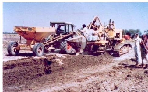
Figure 17: Laying of tile drainage in Sindh
