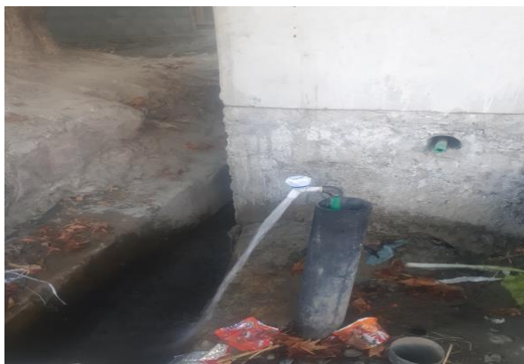
Figure 18: Water tap installed on the corner of water drainage line
