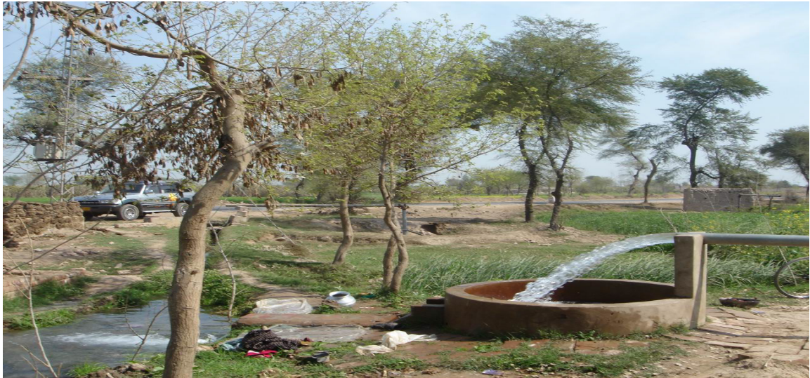
Plate 3: Three tube wells installed about 15 m apart in the LBDC (Lower Bari Doab Canal) command area
